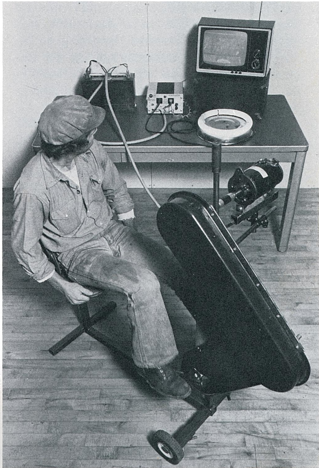
Figure 3-14 Generating electricity with the Energy Cycle
